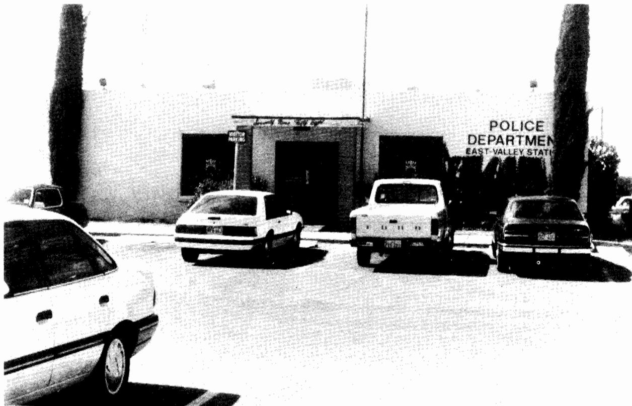
El Paso East Valley substation. Substations in El Paso only house Patrol Operations while Regional Commands are fully self-sufficient police facilities.
