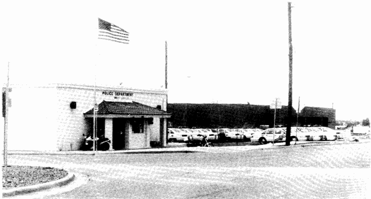
Photo of current Westside substation and future Westside Regional Command Center in background.
